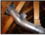
Flue Condition: Satisfactory - The furnace/boiler flue as installed appears to be in satisfactory condition.
